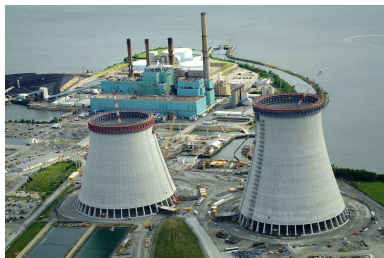
Brayton Point Power Station
